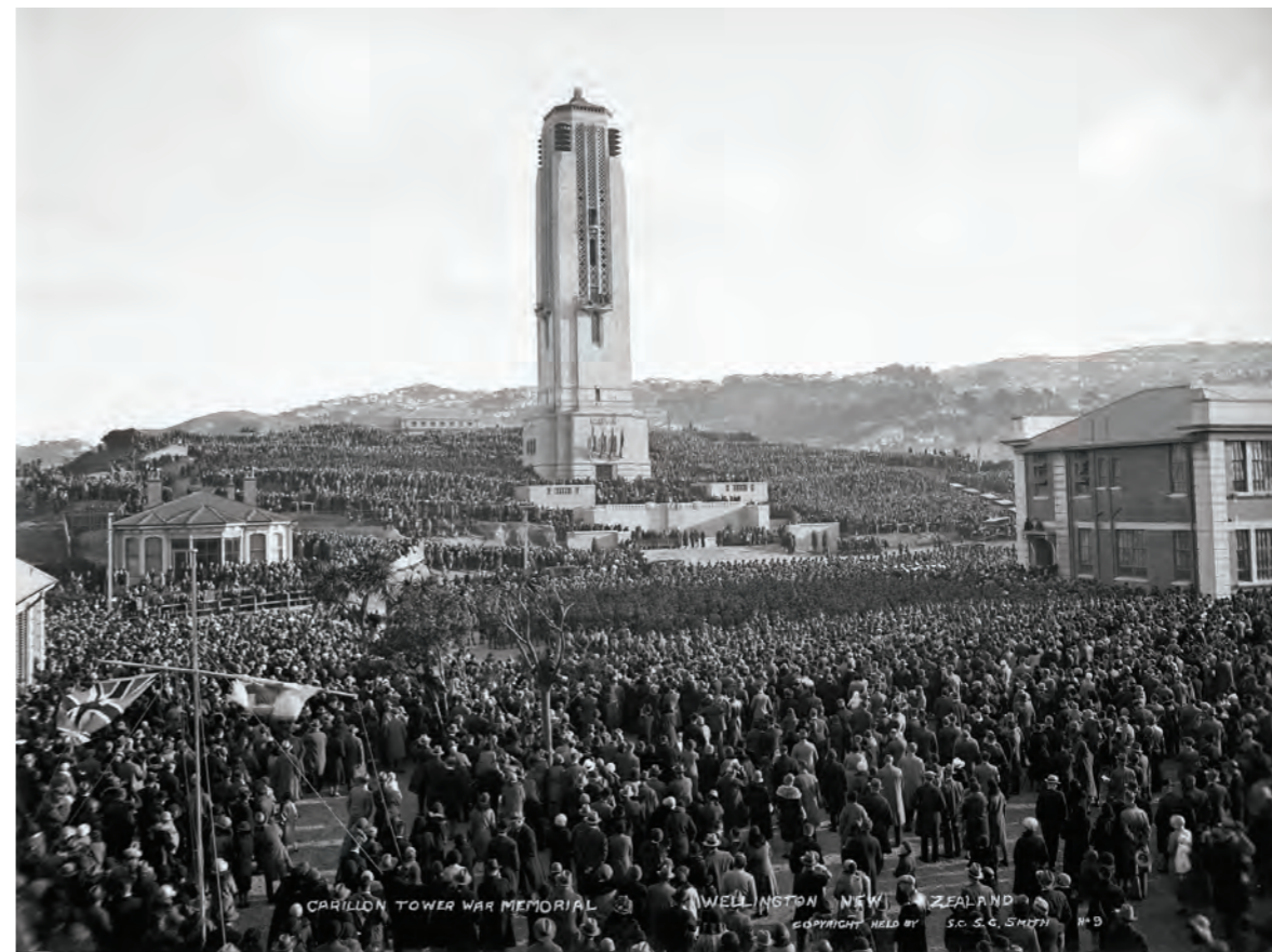
Crowds filled the empty spaces on the hill when the Carillon tower was dedicated on Anzac Day, 25 April 1932.
