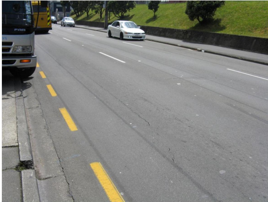
Item 27: longitudinal cracking on existing pavement on RHS of road.
