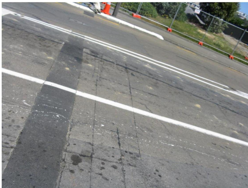
Item 13: water main trench crossing full width of road opposite by-pass road works position. Well-constructed trench repairs.
