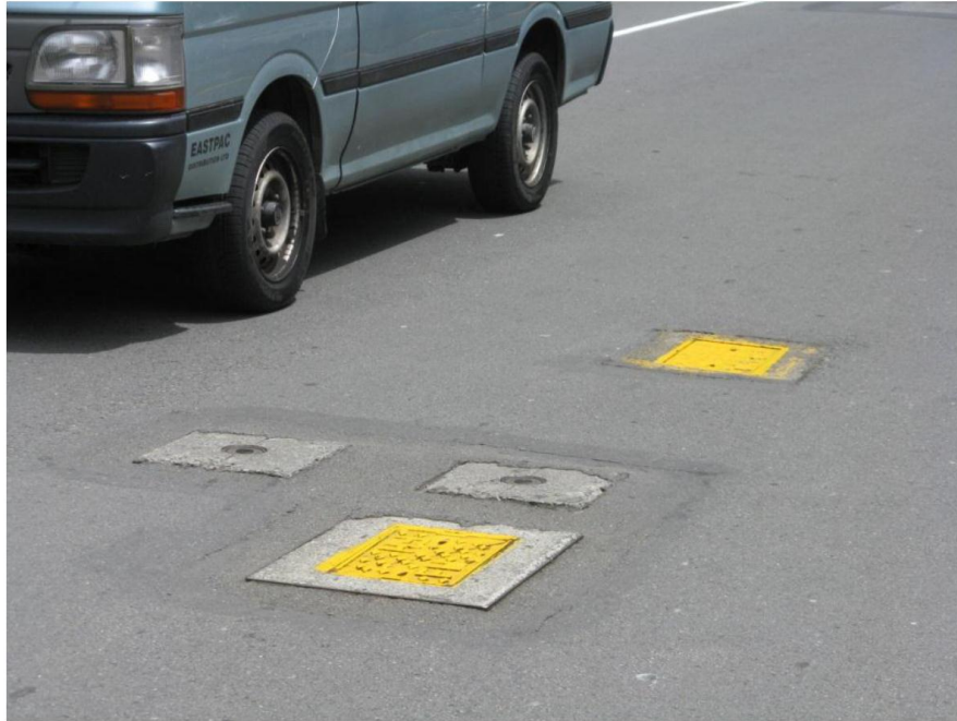
Item 29: Slump around fire hydrant lid
