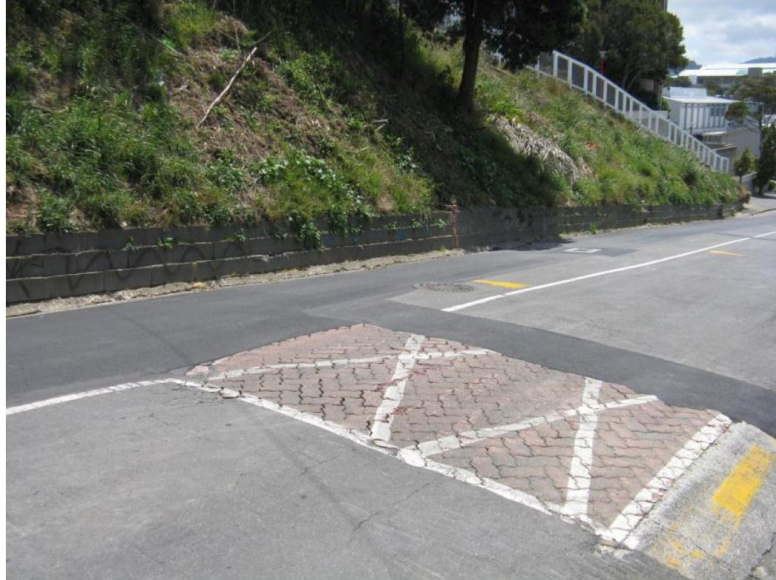
Item 6: Tiles broken on speed hump – probably due to recent stormwater trench works
