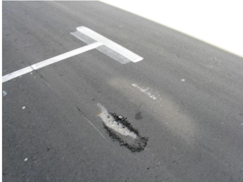
Item 21: Pavement damage / gouge
