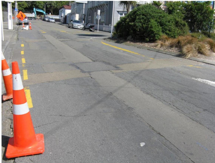
Item 3: Pavement repairs and water main trench (full length of road). Repairs are in good condition.
