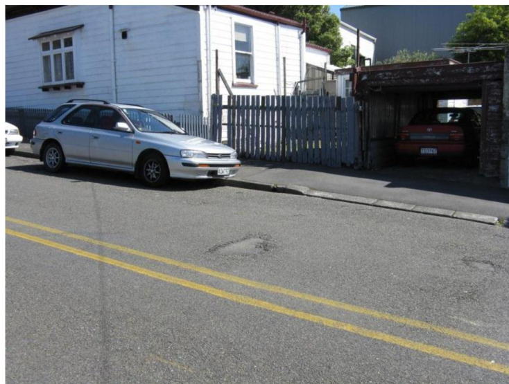
Item 5: Scabbing of existing seal on RHS - multiple small patches
