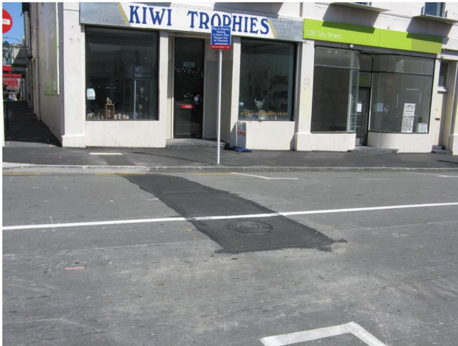
Item 17: Recent trench works - well constructed and no faults
