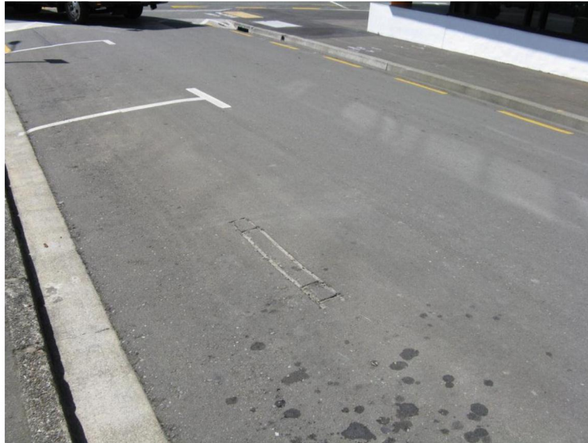
Item 23: Minor seal damage
