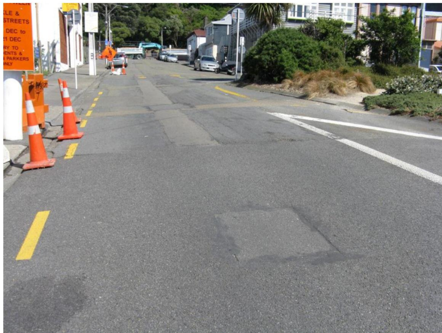
Item 2: Seal joint on Rugby Street and example of older pavement condition and previous repairs
