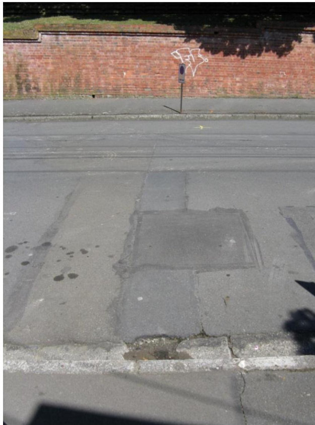
Item 8: Several pavement repairs – joints are in good condition
