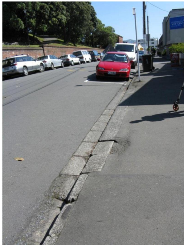
Item 9: Minor slump at driveway to Seventh Day Adventist Church. Existing kerb and channel also broken / cracked.
