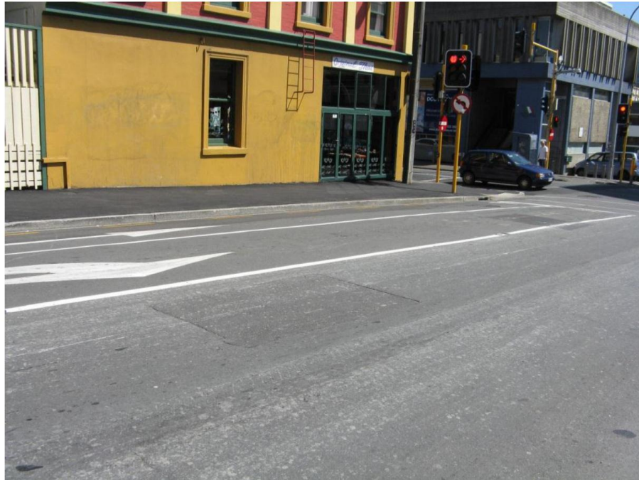
Item 19: minor slump in pavement repair but remains waterproof
