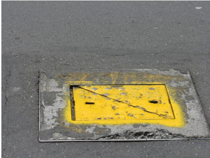
Item 31: broken concrete surround at fire hydrant lid
