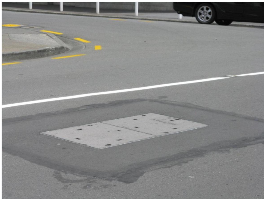
Item 30: well-constructed repair around Telecom lid
