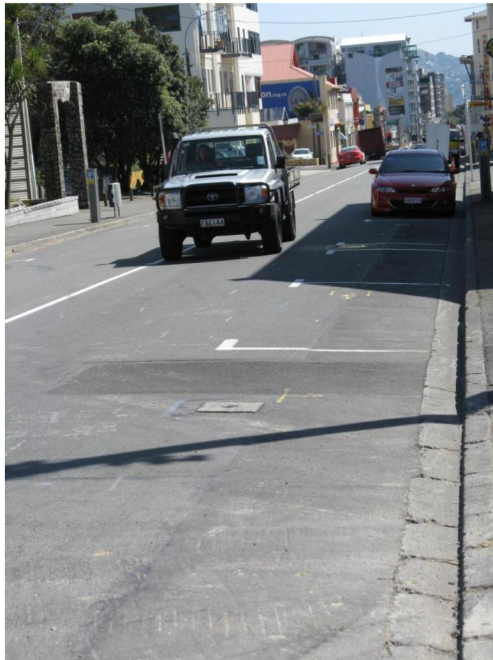
Item 15: pavement repair near coffee shop entrance – seal joints are in good condition. Broken kerb and channel at accessway.
