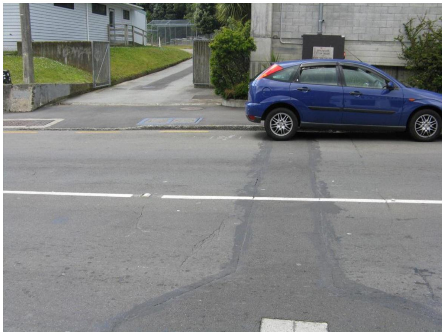
Item 28: lateral cracking on existing pavement adjacent to trench works
