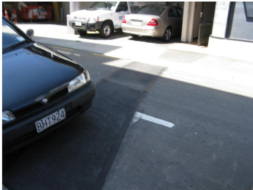
Item 22: Lateral trench repair – well constructed works
