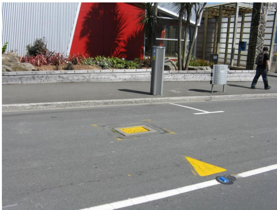
Item 16: pavement subsidence at fire hydrant. Area has already been identified for repair by Council as indicated by yellow markings
