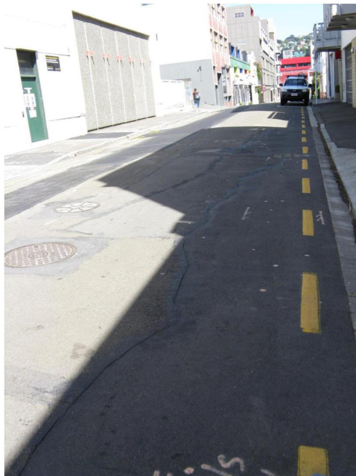
Item 20: Longitudinal cracks in trench repair with poor seal joints
