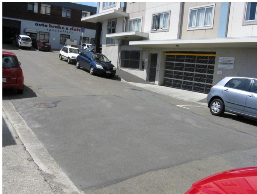
Item 24: Pavement replacement due to recent stormwater works – good shape and condition
