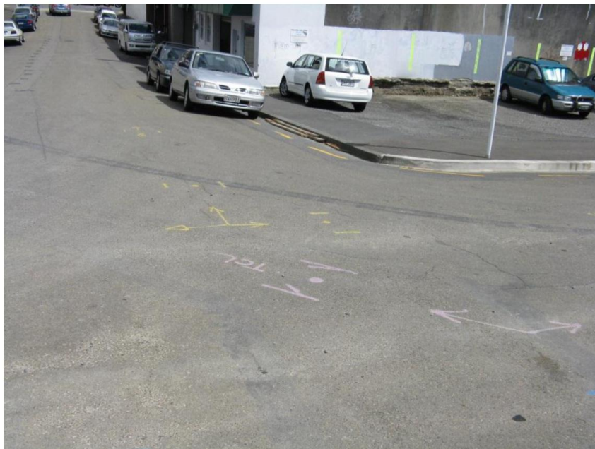
Item 26: Pavement failure - surface damage and potential shallow shear / basecourse problems.
