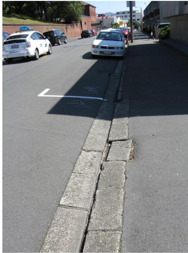
Item 10: Minor pavement and kerb damage at Tasman Street Vet Centre entrance.
