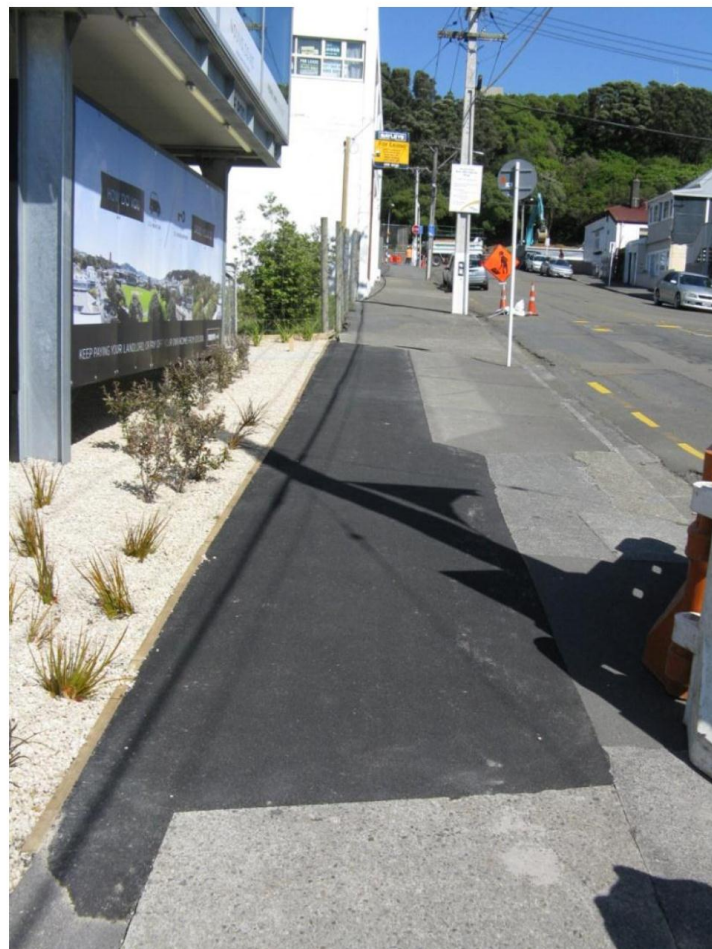
Observation: Footpath repair on LHS (facing uphill). Good condition
