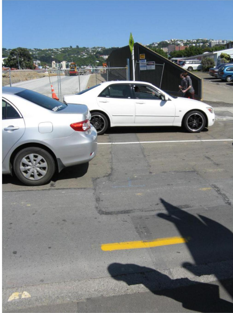
Item 14: minor pavement subsidence at repairs - slight deformation in pavement surface but seal joints are in good condition.
