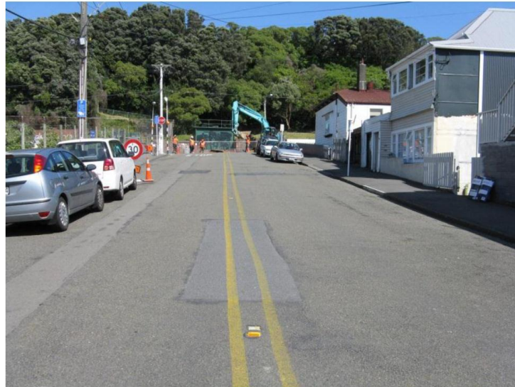
Item 4: Existing pavement repair and water main trench (LHS). Well-constructed works
